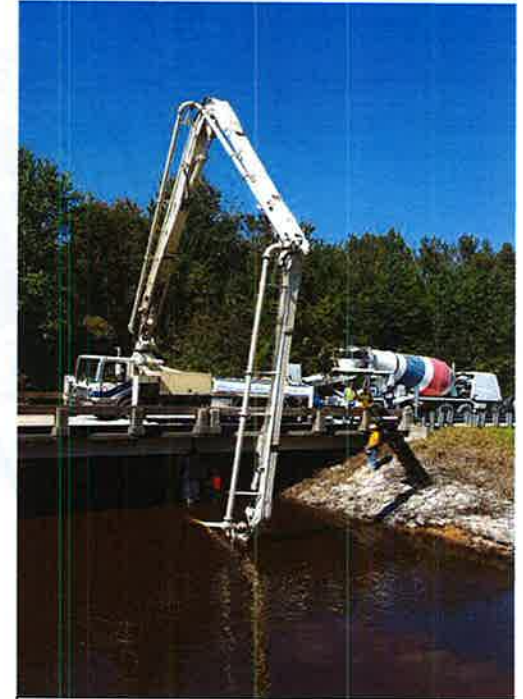
I-95 Bridge Foundation Repairs
