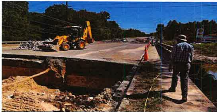
Monticello Road Bridge End Repairs
