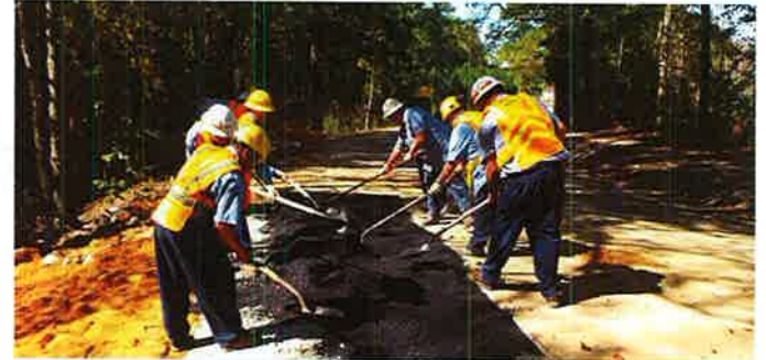
Shoulder and lane repairs
